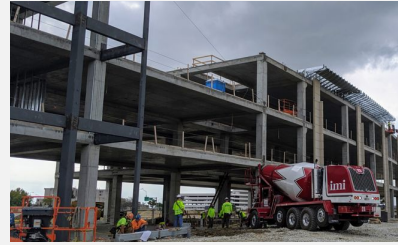
Indianapolis, IN – Infosys Innovation Hub Concrete Producer: Irving Materials CO 2 Saved: 240,000 lbs
