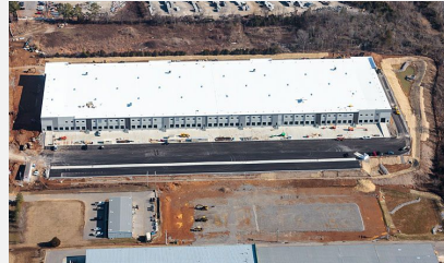
Lebanon, TN – Cedar Creek Distribution Concrete Producer: Irving Materials CO 2 Saved: 140,000 lbs
