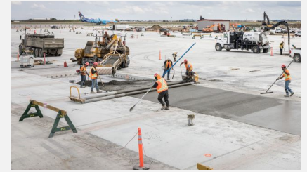
Calgary, AB – East Deicing Apron Owner: YYC Calgary International Airport CO 2 Saved: 352,740 lbs (160 tonnes)
