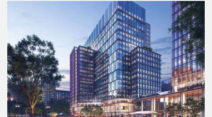
Arlington, VA – Amazon HQ2 Concrete Producer: Miller & Long CO 2 Savings (est.) : 2,500,000 lbs
