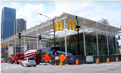
Chicago, IL – McDonald's Flagship Concrete Producer: Ozinga CO 2 Saved: 30,000 lbs
