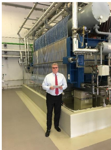
One of three 2MW electrolyzers
